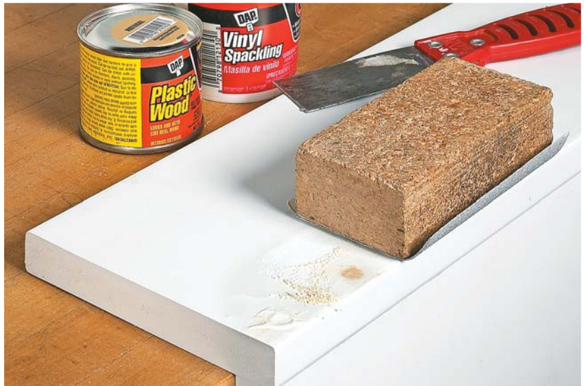
Holes and gouges in PVC lumber are easy to fill using either plastic wood filler or vinyl spackling. Overfill the hole, let the filler harden, and then sand it flush with the surrounding surface. Finish up by applying a coat of primer.
