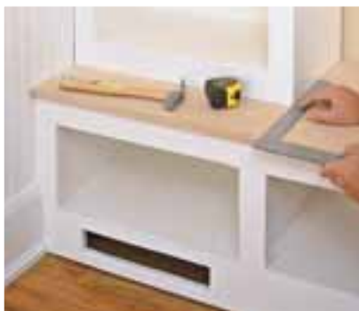
Use a framing square to make sure each tall case is positioned properly before scribing it and before installing it.
