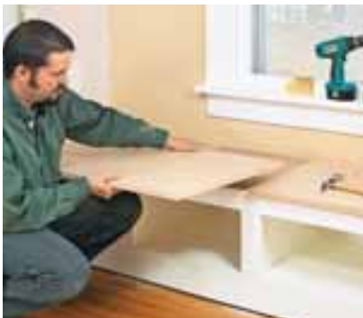
Each seat panel gets trimmed to fit the wall on the back and outside end. The panels should meet tightly at the center.
