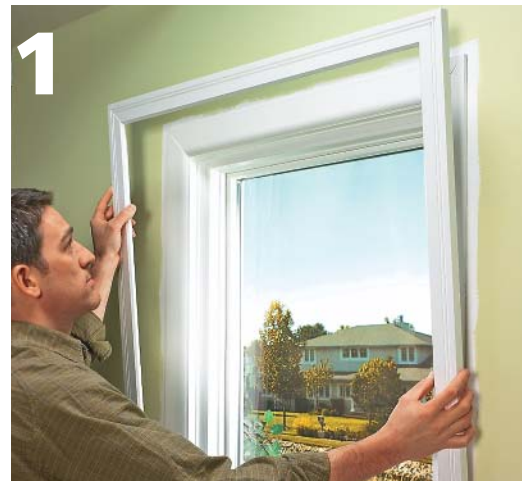
To install the frame, set it over the existing window trim, so the reveal is even all around. Check for gaps (Fig. 2) before nailing the frame in place.
