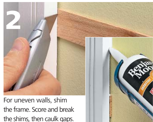
To install the frame, set it over the existing window trim, so the reveal is even all around. Check for gaps (Fig. 2) before nailing the frame in place.
